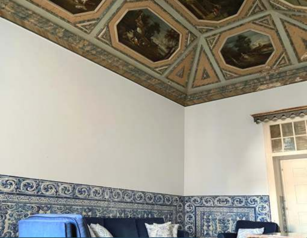
G Panels Room
